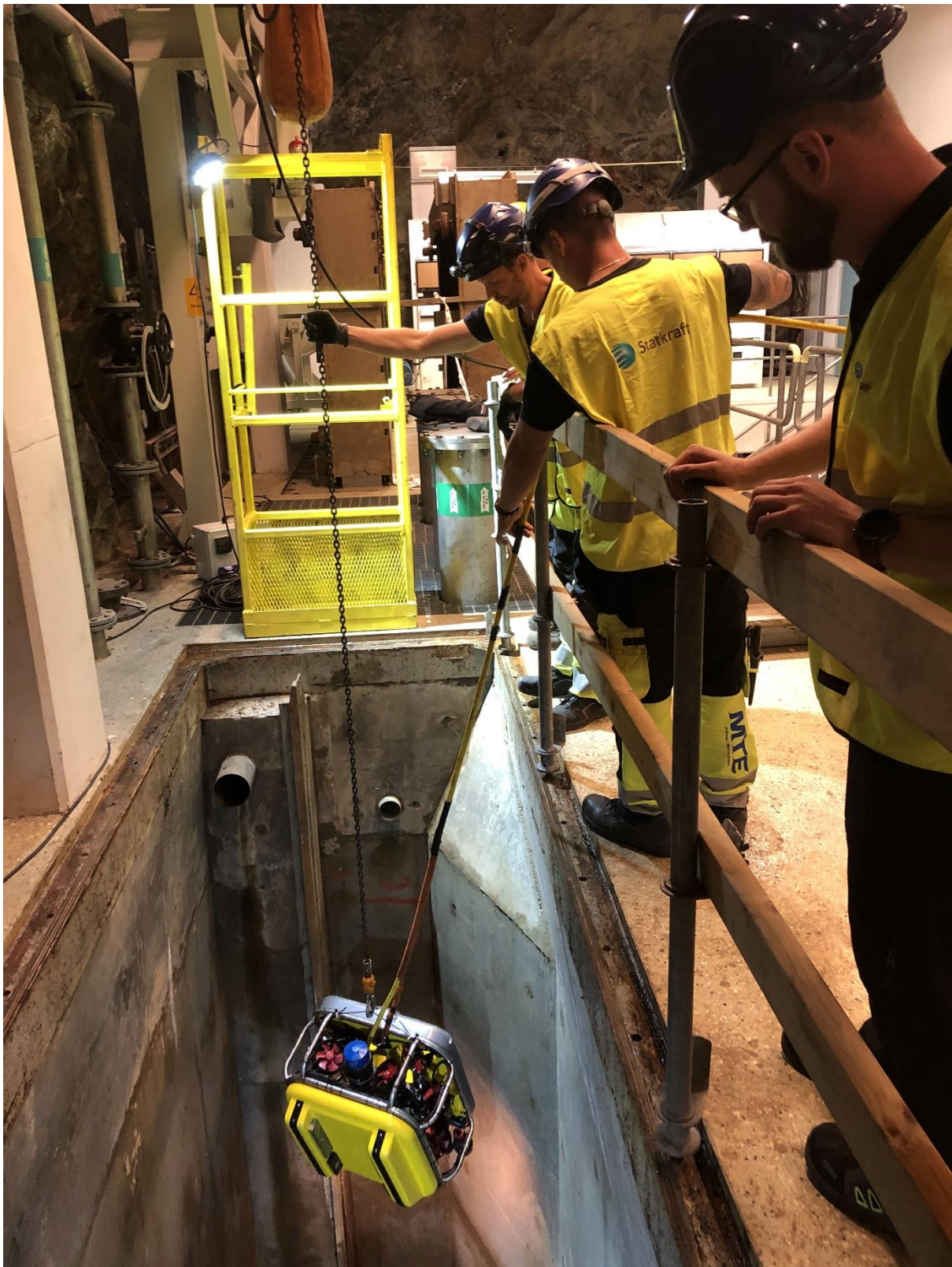
Figure 4. Lowering the ROV into the shaft behind the Turbine.
